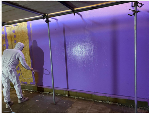
Timber frame wall.
