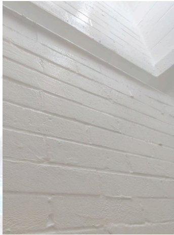
Passive Purple Airtight White Edition retrofit.
