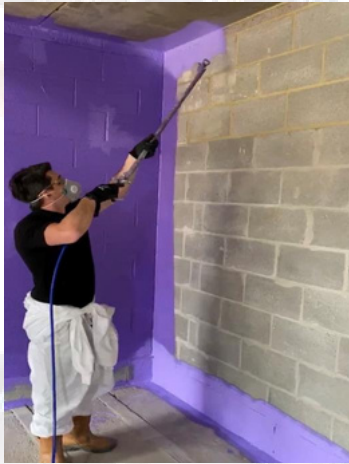
Passive Purple spray install.
