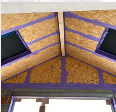
OSB board connections.
