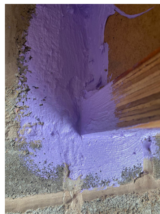
Joist connection on to masonry wall.
