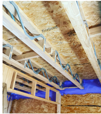
Wall to ceiling connection using Passive Purple Brush.
