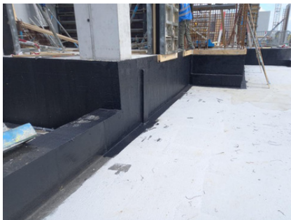
Application on a basement floor
