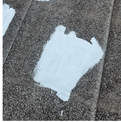
Close up of patching
