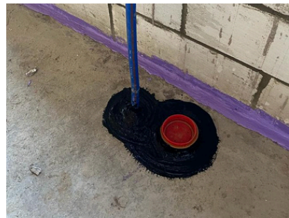
Application around a service penetration
