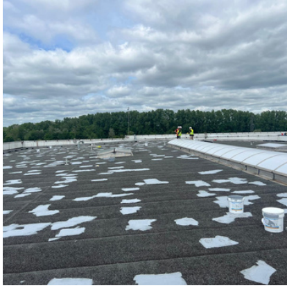
Patching on a roof
