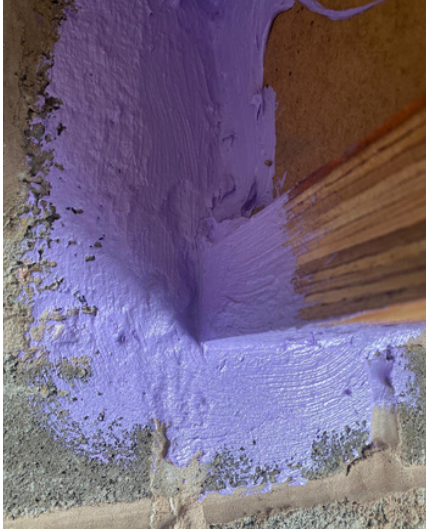
5.1.2 Joist connection into masonry wall
