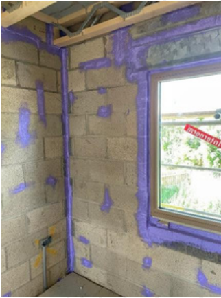
2.2.9. Internal brick connections
