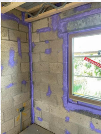
Internal brick connections.
