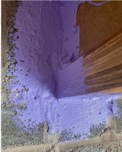
Joist connection into masonry wall
