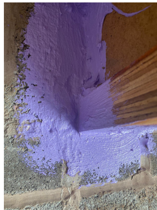
Joist connection on to masonry wall.
