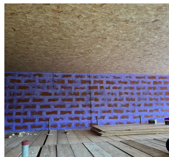
Passive Purple Passivhaus Airtight Sealant applied to wood fibre.
