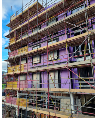
Tower block install.
