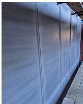
Intelligent Protect install.
