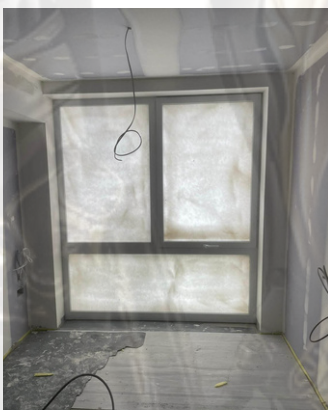
Intelligent Protect install.
