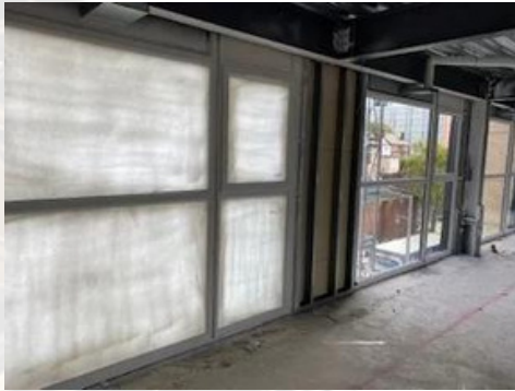
Intelligent Protect install.
