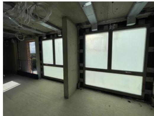
Full temporary protection.
